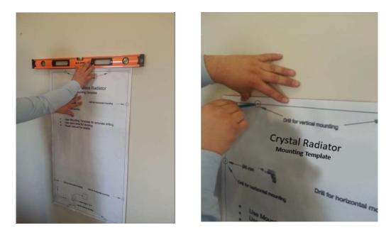
3) Drill the four drilling positions just marked out with the 10 mm drill and following this guide the dowel into the hole .
