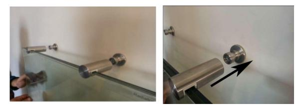
8) Now, slightly tighten the fastening screws attached to the side of the upper glass holders (Part B) with the Allen key that comes with the delivery.
