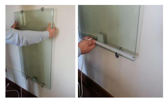
7) Loosely place the two remaining glass holders upon the upper glass edge. While keeping the lower edge of the heating element inside the lower glass holders, move the panel towards the wall until the upper adapter pieces(part A) inserted into the upper glass holders ( part B).
